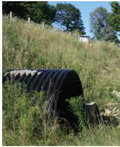
Laminates and coatings have increased the service life of culverts.
