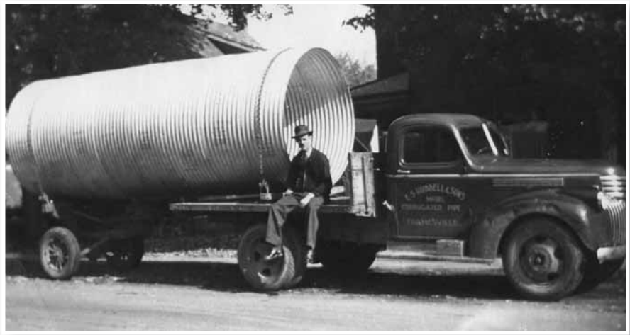
Glen A Hubbell with 9.75m long riveted corrugated steel pipe (circa 1949).
