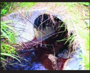
30/2206/1296. This pipe is a 48-inch equalizer/cross drain underneath a two-lane road (route 30) that connects two bogs. At the time of the inspection, there was 10 inches of water flowing toward the east. The pipe is constructed of six sections with polymer-coated bands. All joints were tight and exhibited no signs of leakage.
