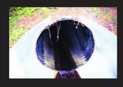
**30/2206/1704.** This pipe is a 24-inch cross drain underneath a two-lane road (Rte 30). The pipe is a 4.5-foot extension on one end of an existing concrete pipe. There was a trickle flow of water at the time of our inspection.
