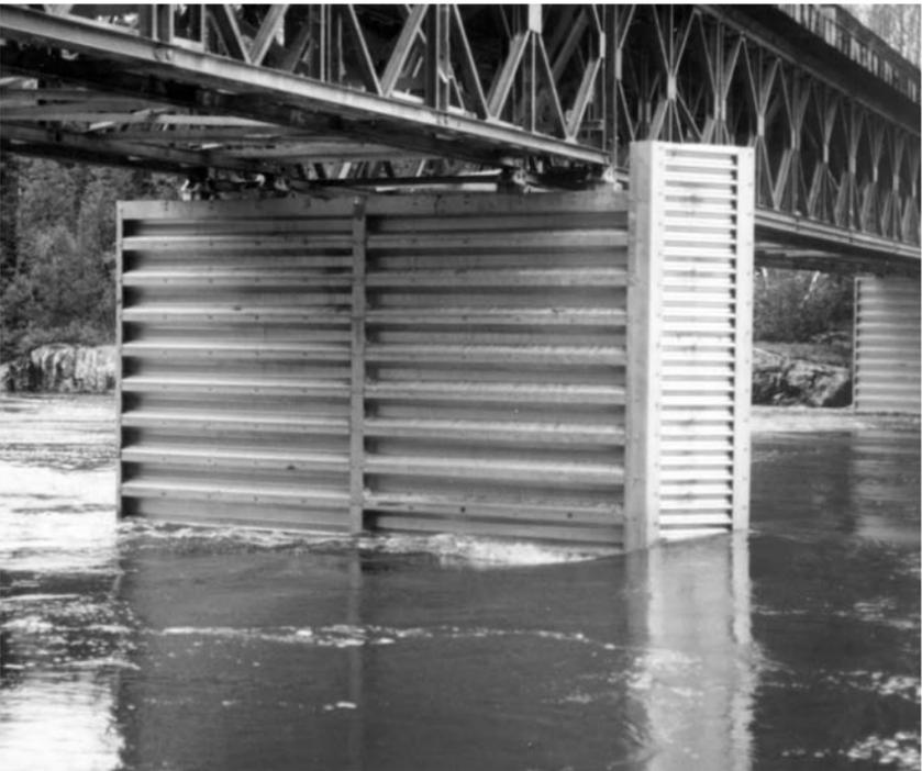
Bridge pier uses bin type retaining wall components.
