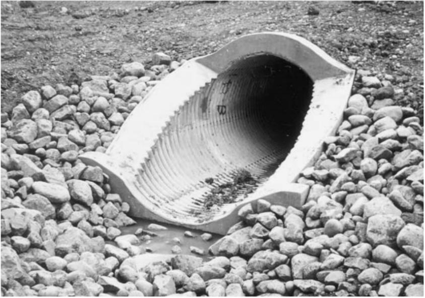
Structural plate CSP with concrete end treatment.
