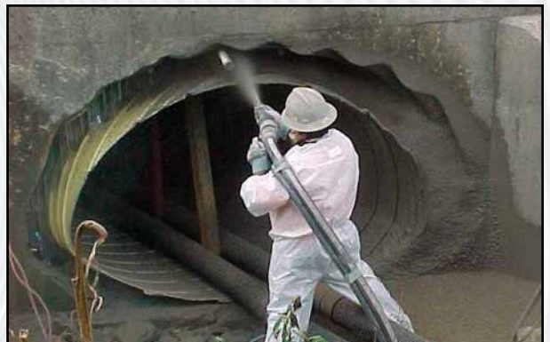
HEADWALL GUNITE INSTALL
