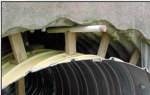
VENT THROUGH HEADWALL
