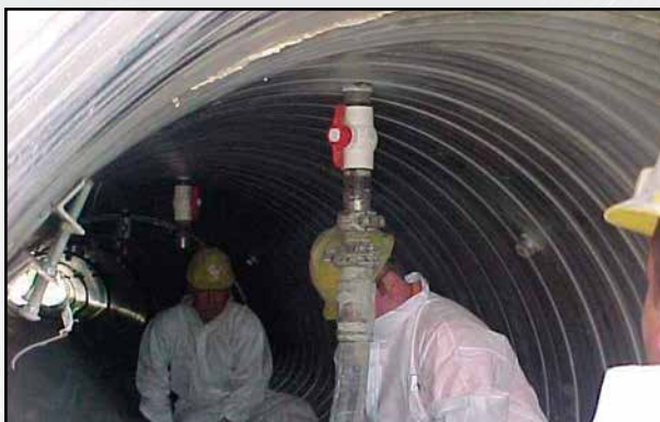
GROUT PORT – LAST LIFT
