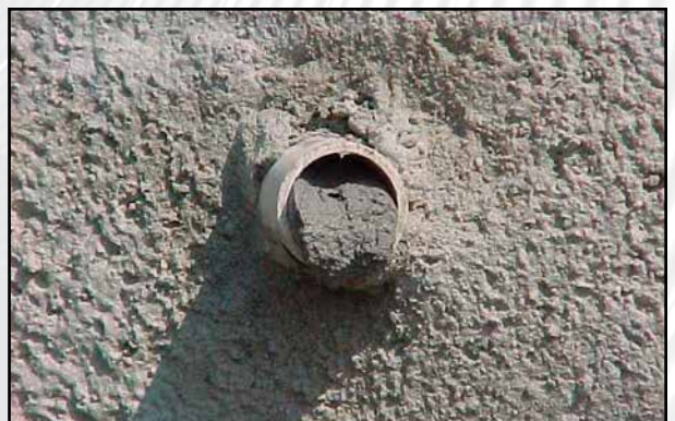
GROUT THROUGH VENT
