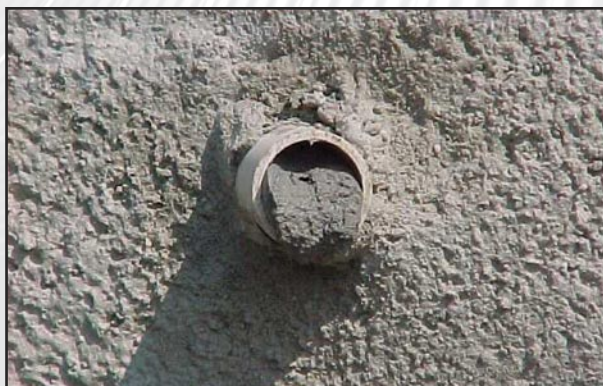
GROUT THROUGH VENT
