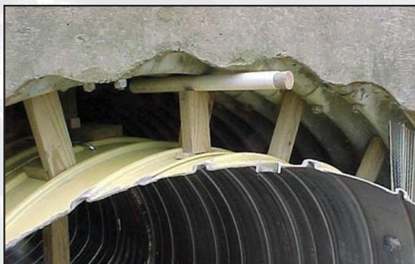
VENT THROUGH HEADWALL
