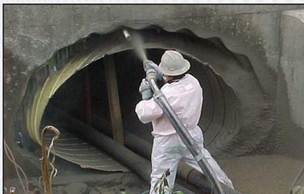
HEADWALL GUNITE INSTALL
