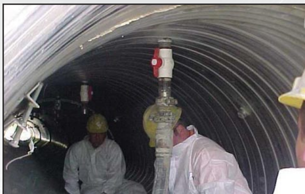
GROUT PORT – LAST LIFT
