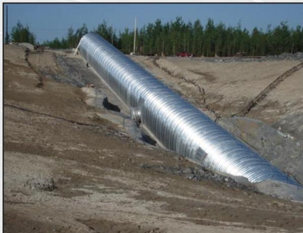
CLAY OVERBURDEN STRIPPED AWAY TO ALLOW INSTALLATION OF 6320 MM SPAN X 5630 MM RISE X 162 M LONG DEEP CORRUGATED STRUCTURAL PLATE ARCH MINE PORTAL
