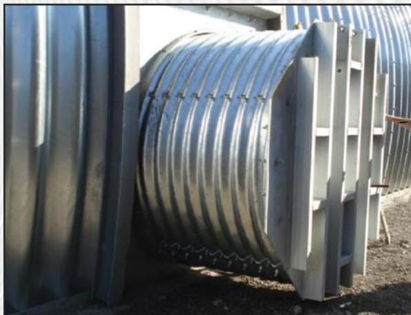
THREE PERSON SAFETY STATION OF 2120 MM DIA. STRUCTURAL PLATE CORRUGATED STEEL PIPE (SPCSP) WITH REINFORCED BULKHEAD AND STIFFENER CHANNELS
