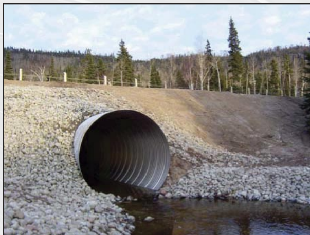
EMERGENCY REPLACEMENT FLOODED BOX CULVERT WITH CSP
