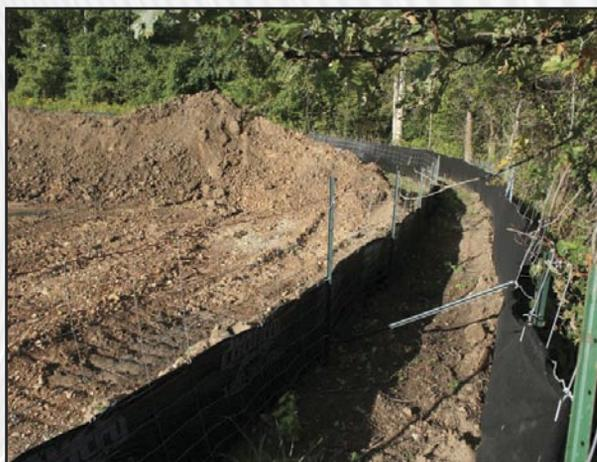
CLÔTURE DE CONTRÔLE DES SÉDIMENTS ET DE L'ÉROSION POUR LA PROTECTION DES TERRES HUMIDES DU PARC INDUSTRIEL DE HANLON CREEK PENDANT LA CONSTRUCTION
