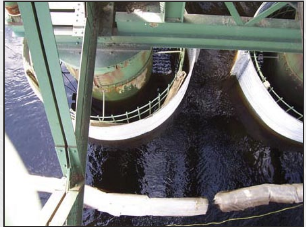
CAISSONS & REINFORCING STEEL IN PLACE
