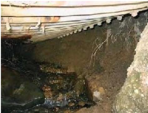
Large Void at Invert\*<sup>3.2</sup>
