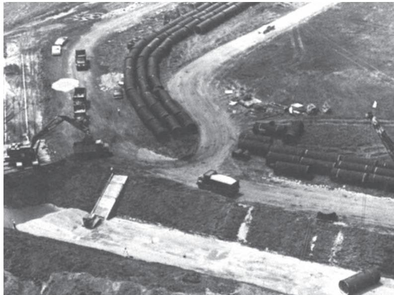
*Philadelphia Airport, 16 x 26mm fiber-bonded, full bituminous coated and full paved CSP with semi-corrugated bands with O-ring gaskets, provides storm drainage for airport— 5800 m of 2000mm, 2200mm, 2400mm, 2700mm diameters, 14 - 16 gauge, 2 - 3m of cover.*
