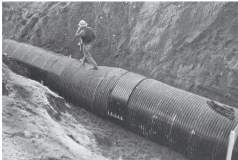
*Increasers are easily fabricated for correct field location.*
