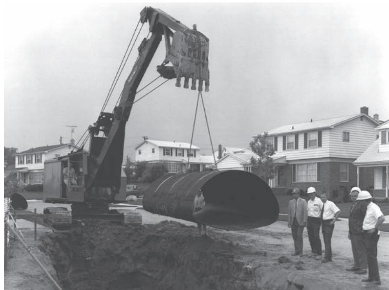
*Pipe-arch sewer installation in a residential area satisfying minimum headroom requirement; however it has adequate capacity and strength.*
