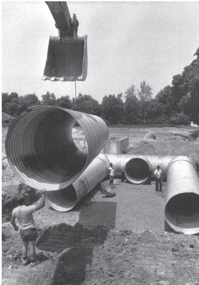
*Installing 1,800mm diameter CSP to be used as an underground detention chamber for stormwater runoff.*
