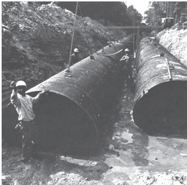
*Storm Sewer installation involved 1300 m of full bituminous coated full paved pipe arch.*
