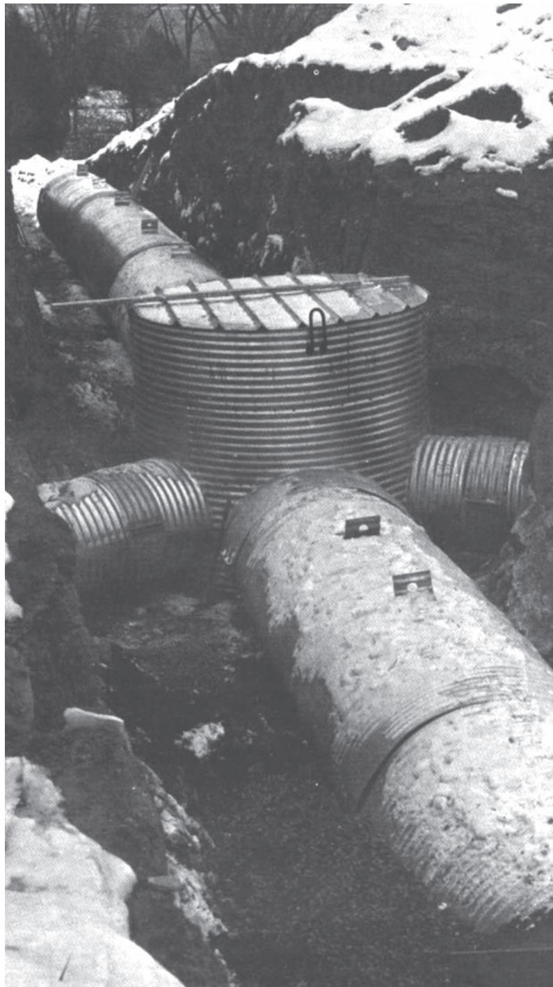
*Fabricated fittings are hydraulically superior.*
