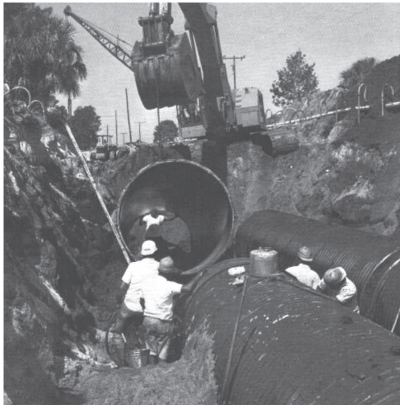
*Smooth-lined CSP storm sewer being installed.*
