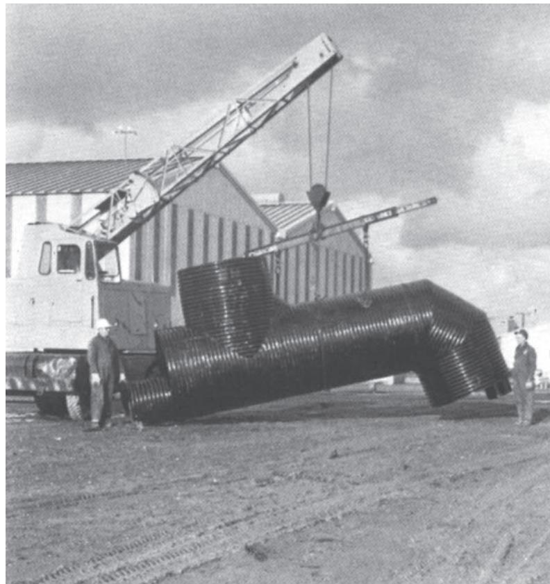
*Combination increaser, manhole and elbow in one length of pipe.*
