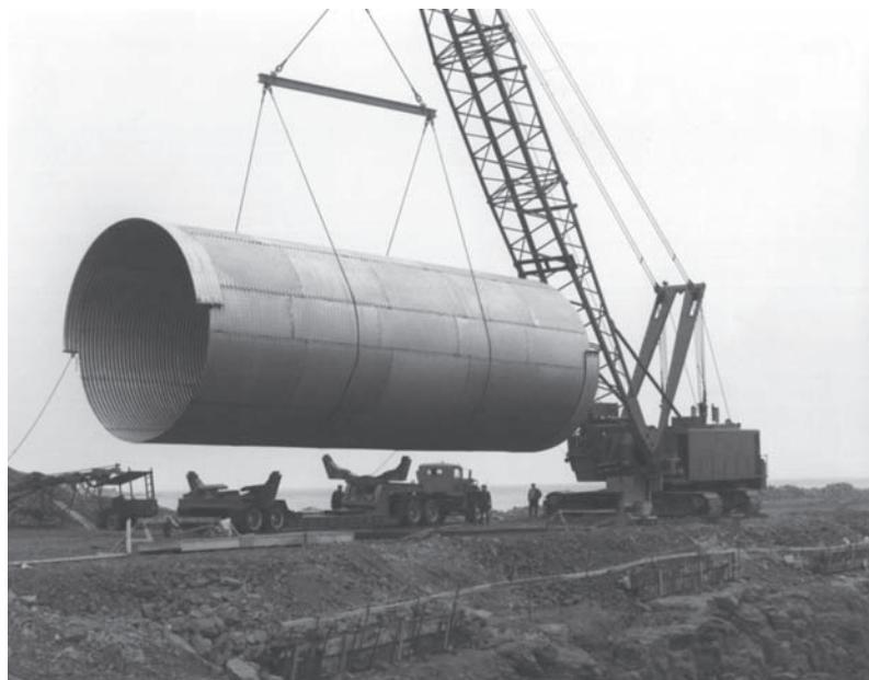
*Large diameter structural plate pipe for handling high volumes of runoff.*
