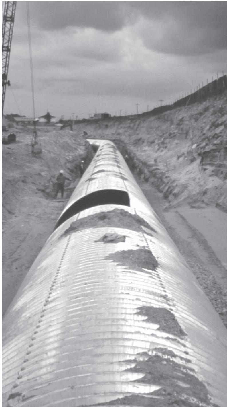
*CSP Sewer designed for very wide trenches.*
