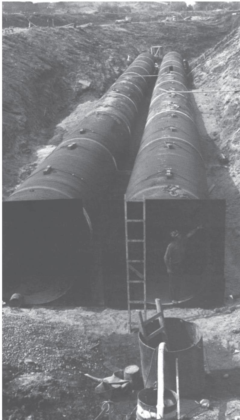
*Large diameter structures installed in difficult trench conditions using the advantage of long lengths.*
