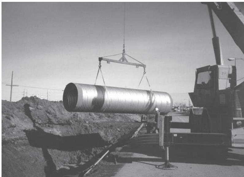
*Exterior coatings are protected during installation by use of lifting lugs or slings.*
