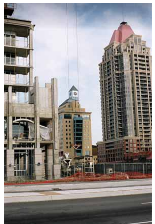
One Park Tower under construction, and the Clock Tower Mississauga City Hall.
